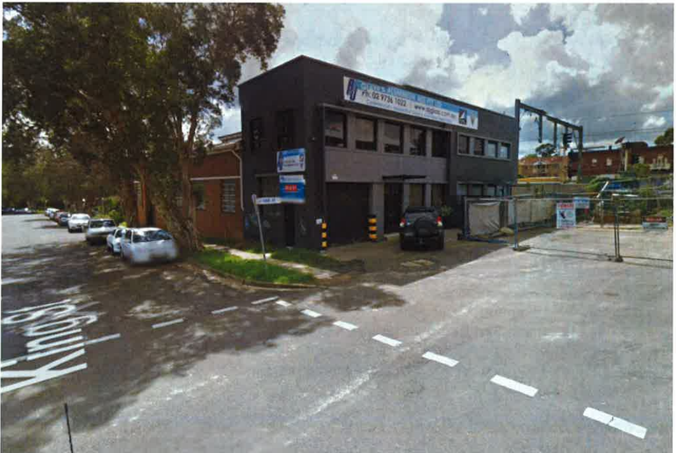
Figure 2: View of subject site from intersection of King Street and Victoria Avenue facing north-east
